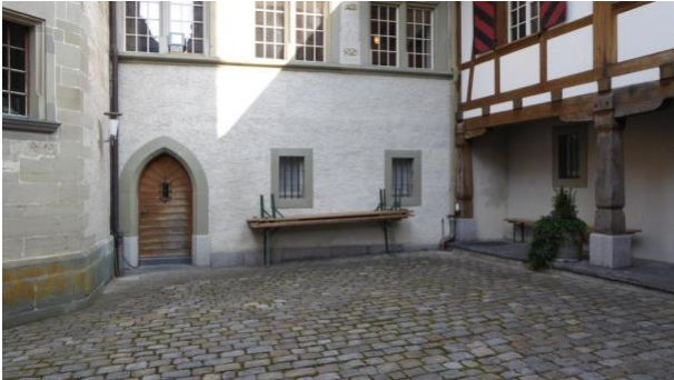
Figure 5: Behind this wooden door in the castle courtyard lies the cell wing, which can be used for the exhibition.
